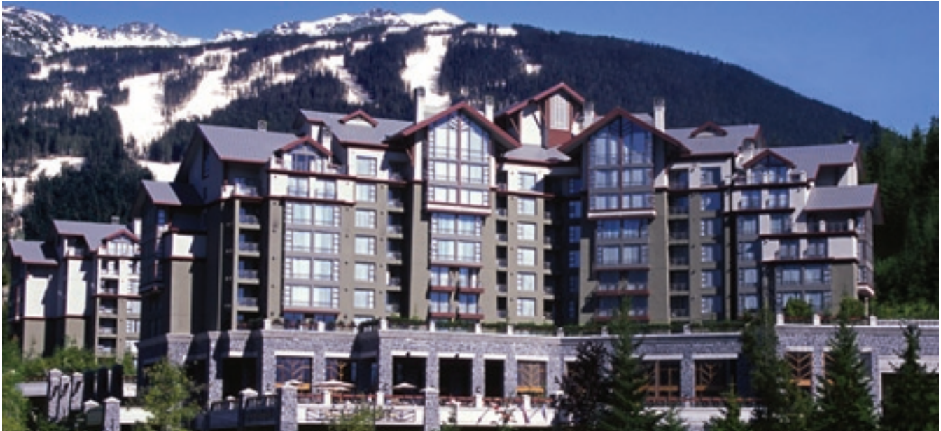
Retractable screens help achieve thermal comfort and energy savings. (Photo courtesy of the Westin Resort & Spa, Whistler, BC.)
