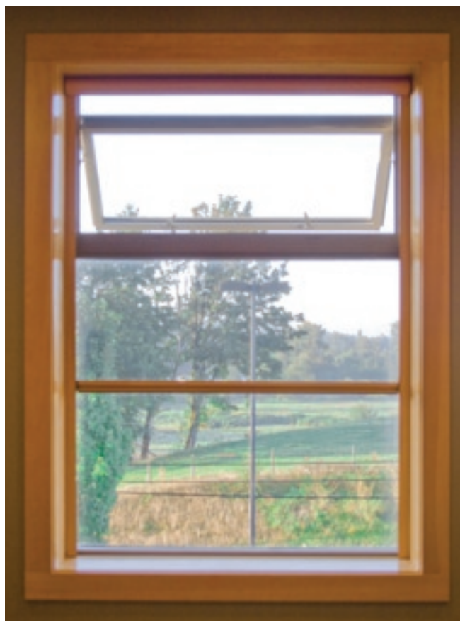
Manually retractable screens can be used in ventilating windows and egress doors. (Photo courtesy of Phantom Screens.)
